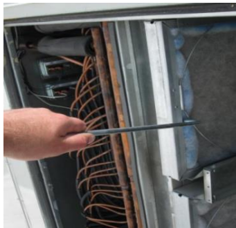
Figure 2. Use Door Arm to Pull Out Filters
