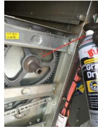
Figure 6. Lubricate Outside
