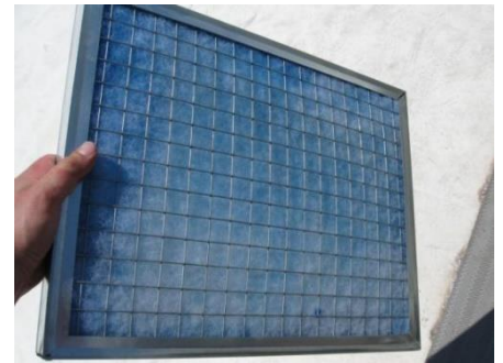
Figure 3. Remove and Replace Filters
