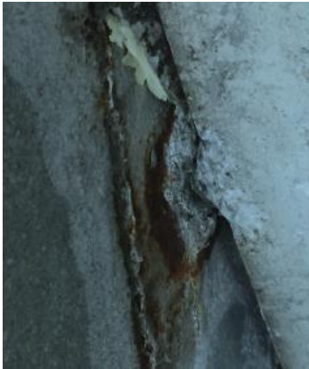
Figure 4. Look for Rust
