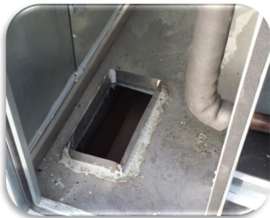
Figure 1. Pipe Chase inside FLō unit before piping has been installed.
