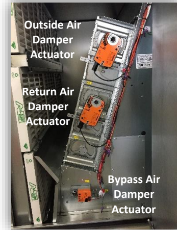
Figure 3. Damper Assembly and Actuators
