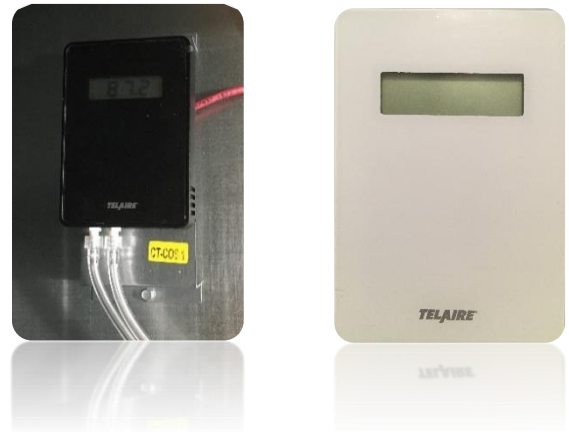
Figure 3. CO2 sensor located inside unit
