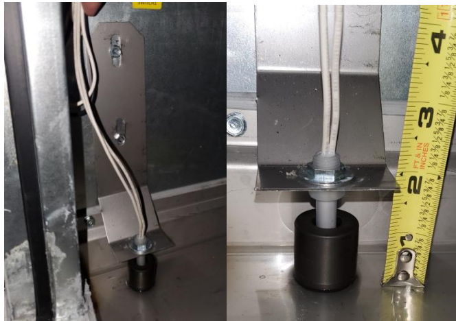
Figure 2. Float Switch Mounting Position
