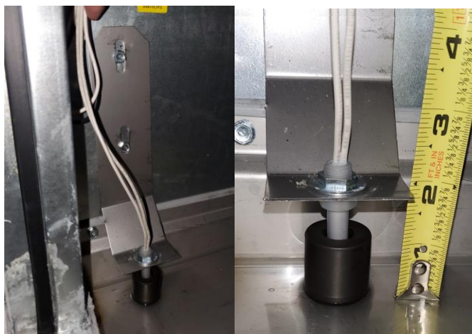
Figure 2. Float Switch Mounting Position
