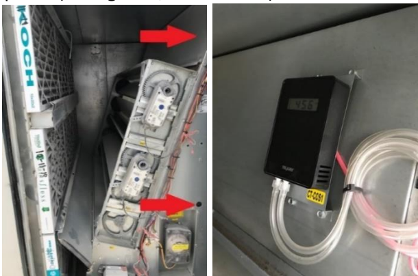
Figure 2. CO2 sensor location inside the unit
