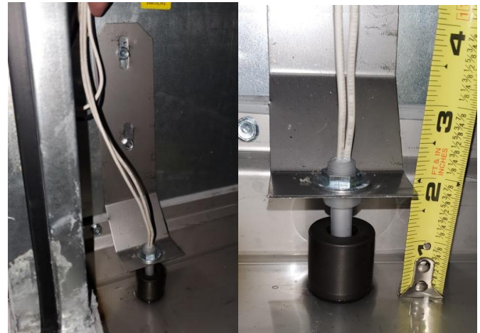
Figure 2. Float Switch Mounting Position
