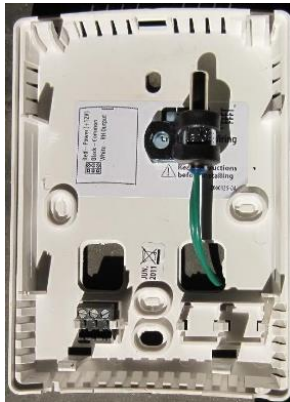
Figure 5.3. 501-1125 Temp Sensor Mounting Position In RH
