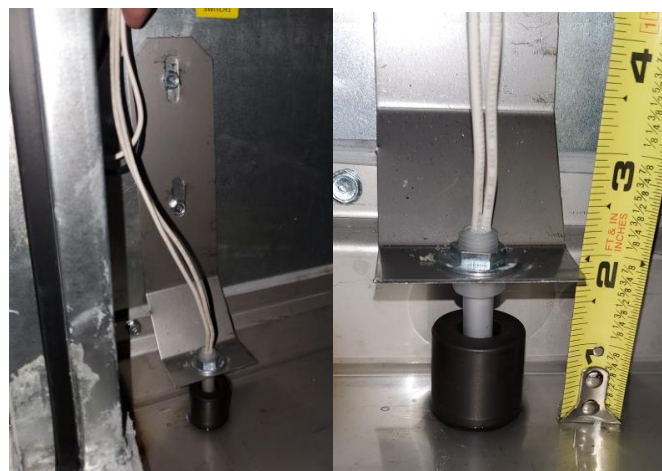
Figure 2. Float Switch Mounting Position
