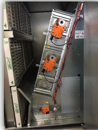
Figure 3. Damper Assembly and Actuators
