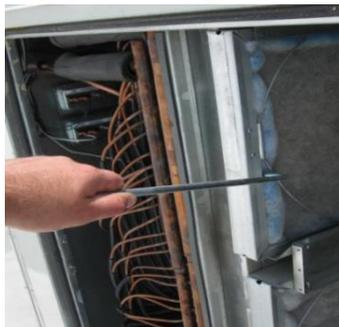
Figure 2. Door Bracket to pull Filter
