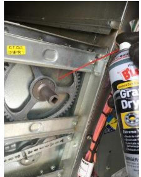
Figure 6. Lubrication of Damper Gear
