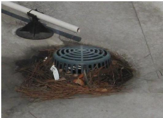
Figure 7. Clogged Roof Drain
