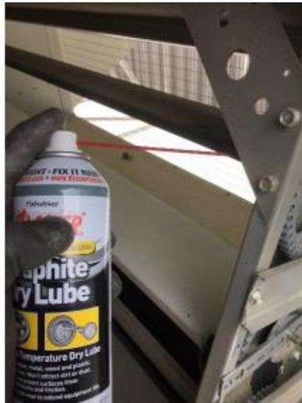
Figure 5. Graphite Lubricant
