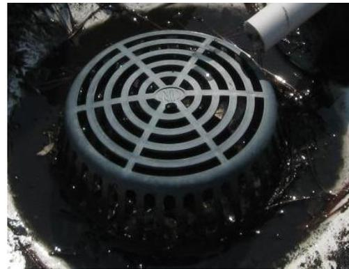
Figure 8. Clean Roof Drain
