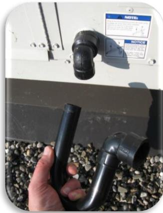
*Figure 11. Factory Provided P-Trap Installation*
