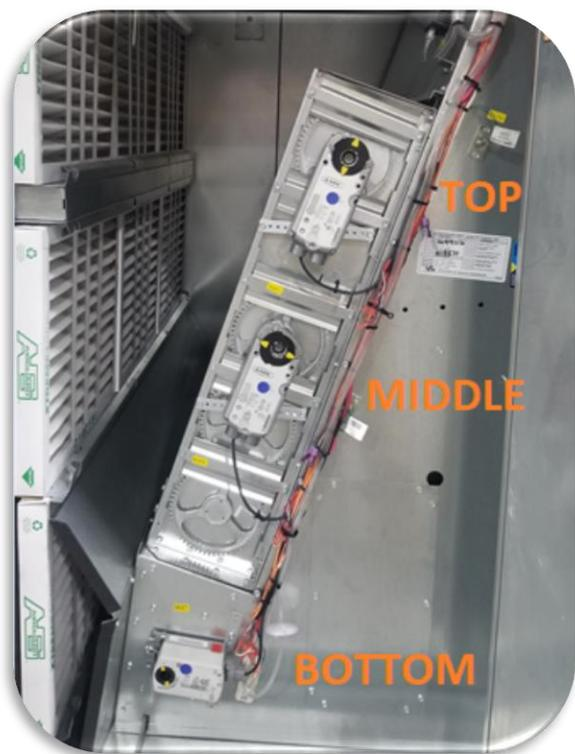
Figure 17. MPU Damper Assembly
