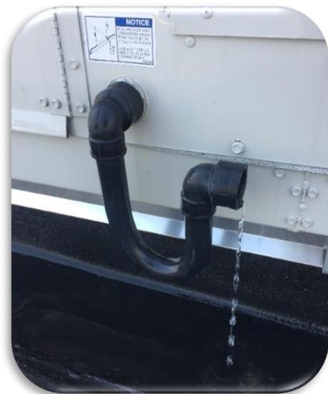
Figure 10. Factory P-Trap Installed
