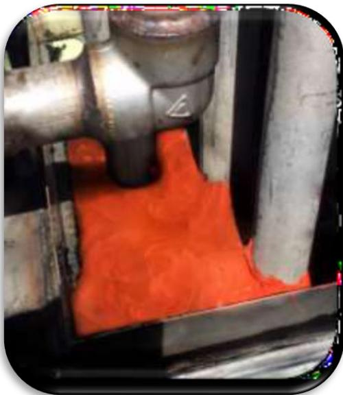
Figure 15. Clean, Sealed Pipe Chase
