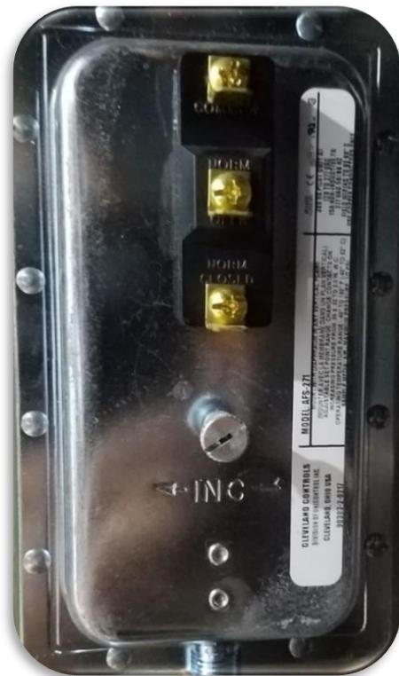
Figure 22. Clogged Filter Switch
