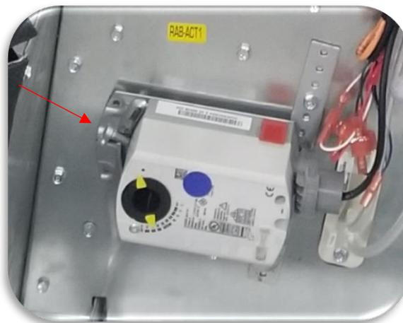
Figure 19. BAD Adjustment Screw Location
