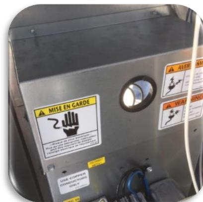
Figure 24. High Voltage Entry Point
