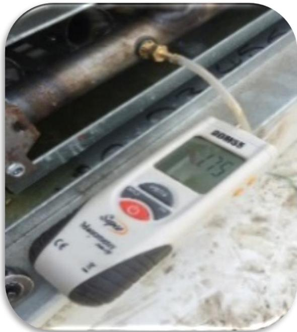
Figure 29. Manometer Connected to Gas Port
