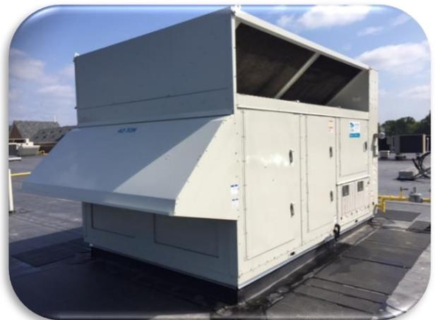
*Figure 2. Flō Large Multi-Path Unit (26 and 31-70 Tons)*
