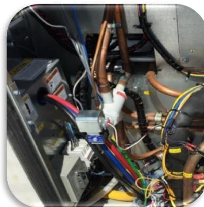
Figure 25. High Voltage Wiring Through Entry Point
