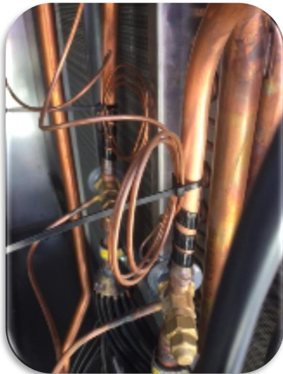
*Figure 13. Secured Capillary Tubes*
