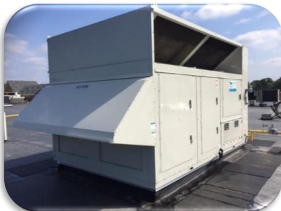
Figure 6. Large Unit - Open Air Hood
