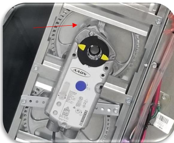
Figure 18. OAD & RAD Adjustment Screw Location
