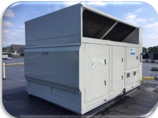
Figure 5. Large Unit - Closed Air Hood
