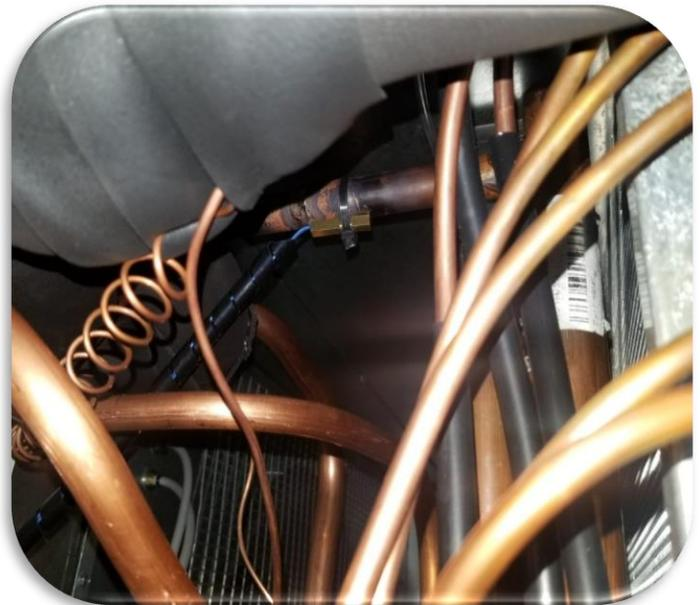
Figure 16. Reclaim Temp Sensor Installation
