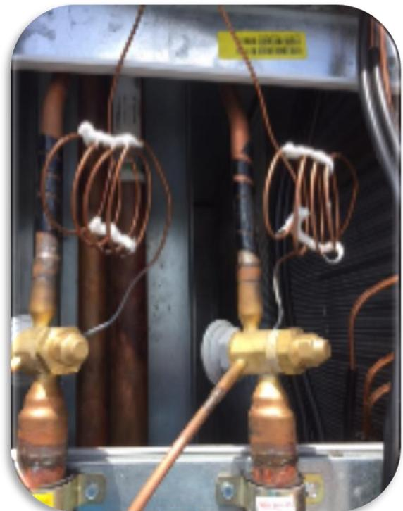
*Figure 14. Capillary Tubes at Start-Up*
