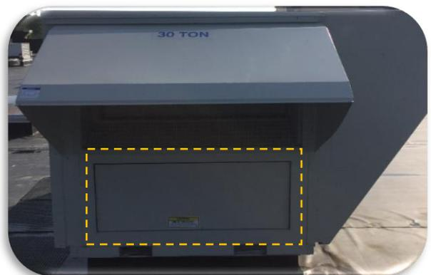
Figure 7. Small Box Barometric Relief Damper
