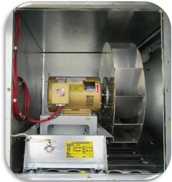
Figure 21. Supply Fan Compartment
