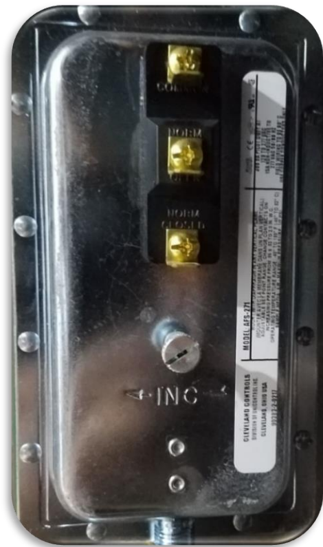
Figure 1. Clogged Filter Switch
