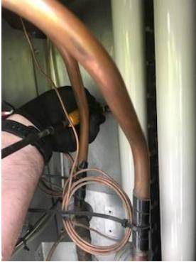
Figure 22. Blower Bracket Screw Removal
