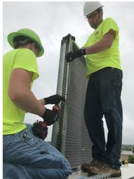
Figure 26. Heat Reclaim Bracket Removal/Installation
