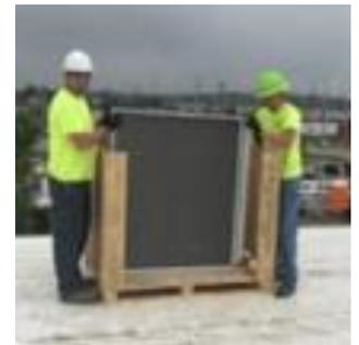
Figure 7. Remove Coil from Crate
