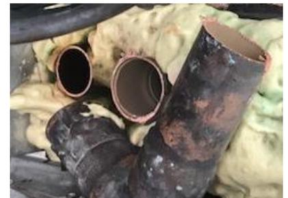
Figure 13. Cut Refrigerant Piping
