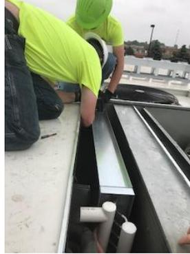
Figure 23. Heat Reclaim Coil Rear Bracket Screw Removal
