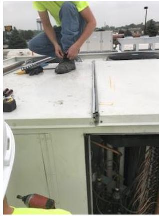
Figure 16. Roof Cap Removal
