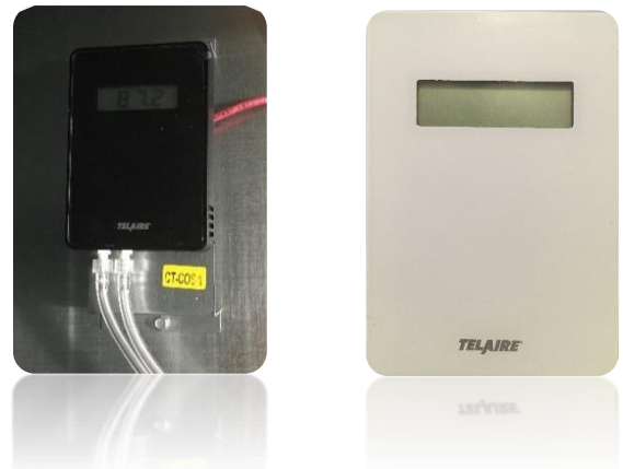
Figure 4. CO2 sensor located inside unit
