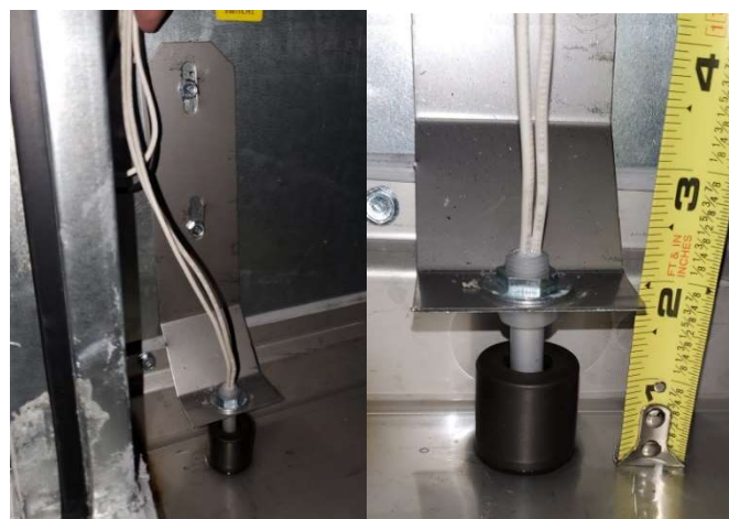
Figure 2. Float Switch Mounting Position
