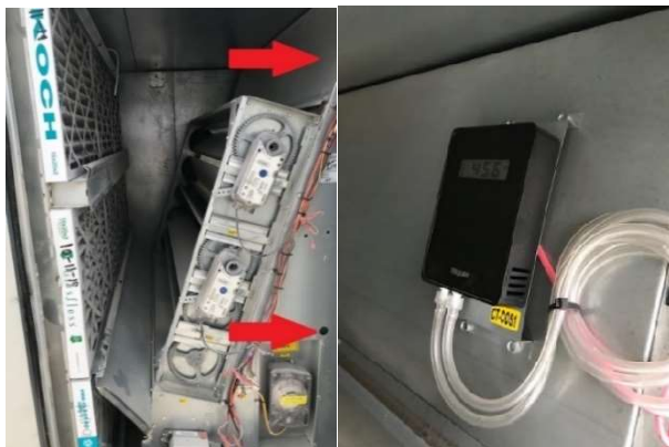
Figure 3. CO2 sensor location inside the unit
