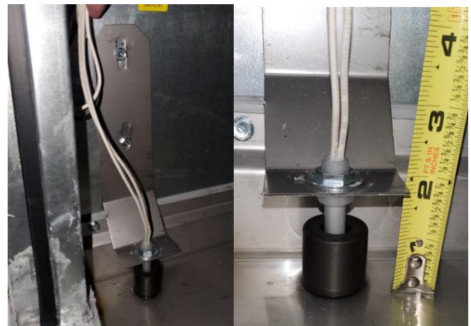
Figure 2. Float Switch Mounting Position
