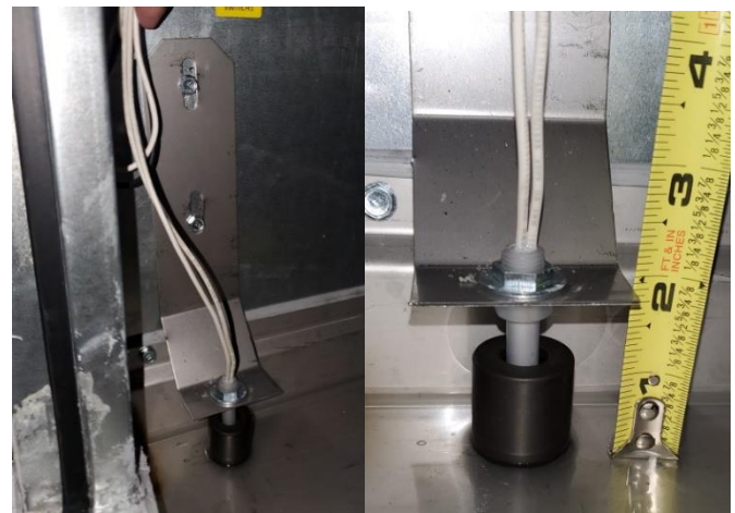
Figure 2. Float Switch Mounting Position
