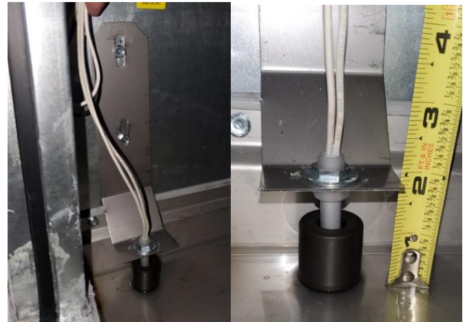
Figure 2. Float Switch Mounting Position
