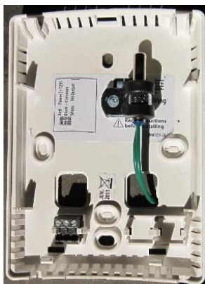
Figure 5.3. 501-1125 Temp Sensor Mounting Position In RH
