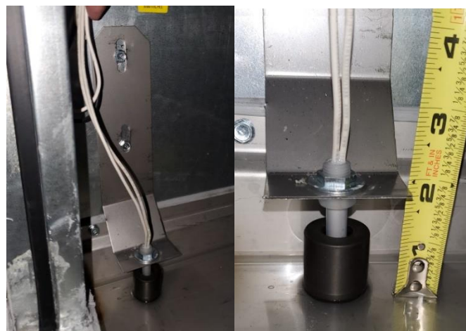
Figure 2. Float Switch Mounting Position
