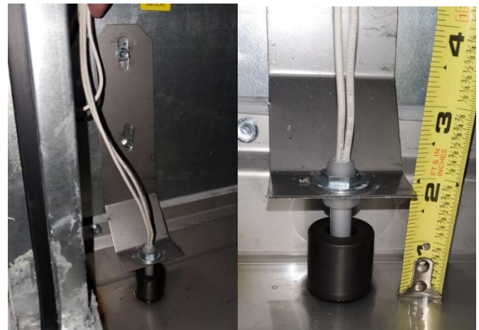
Figure 2. Float Switch Mounting Position
