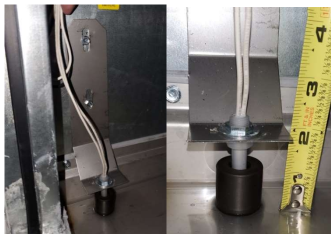
Figure 2. Float Switch Mounting Position
