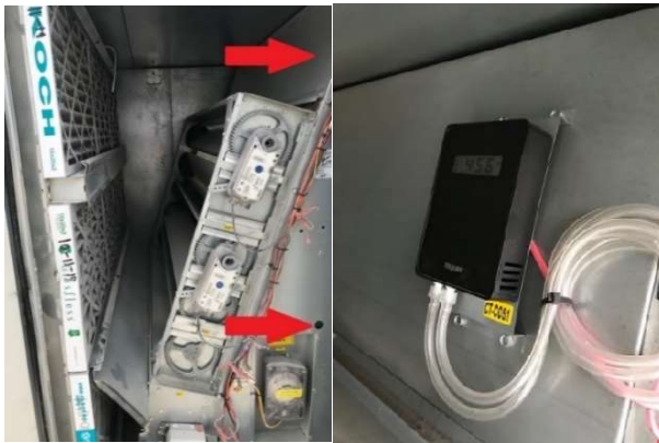
Figure 3. CO2 sensor location inside the unit
