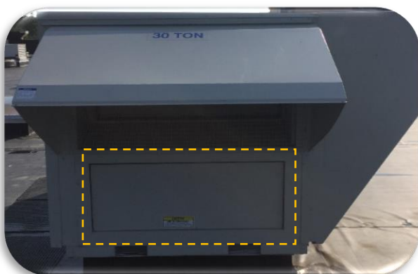
Small Box Barometric Relief Damper
