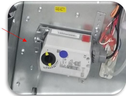
BAD Adjustment Screw Location
