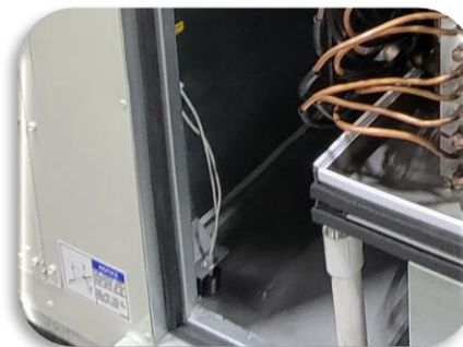
Drain Pan Float Switch
