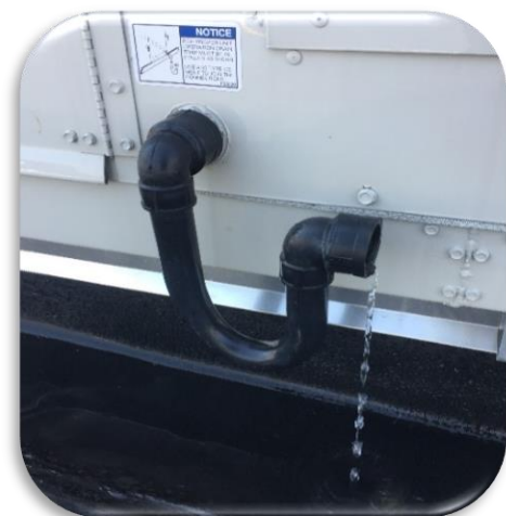
P-Trap Installed
