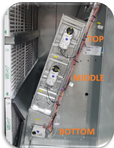
MPU Damper Assembly
