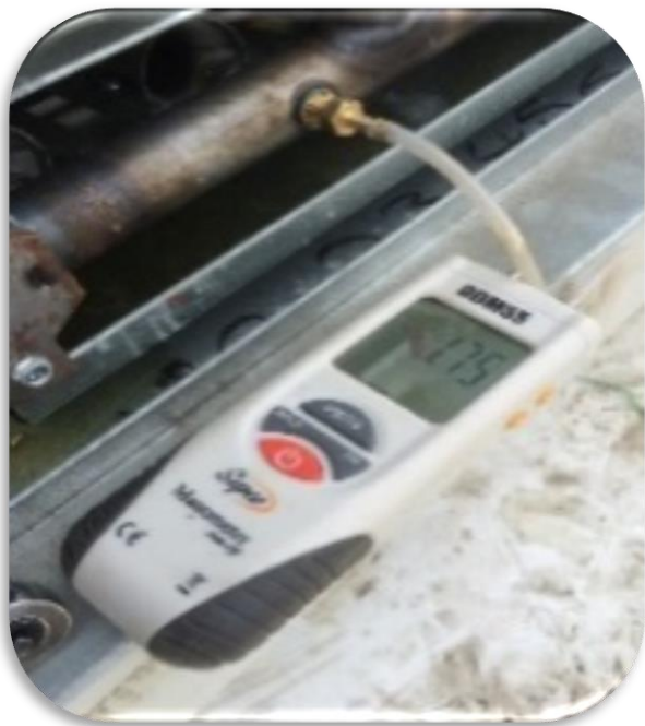
Manometer Connected to Gas Port
