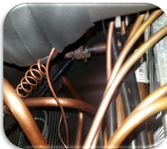
Reclaim Temp Sensor Installation
