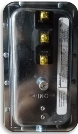
Clogged Filter Switch
