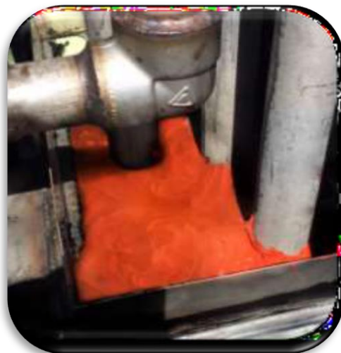
Clean, Sealed Pipe Chase
