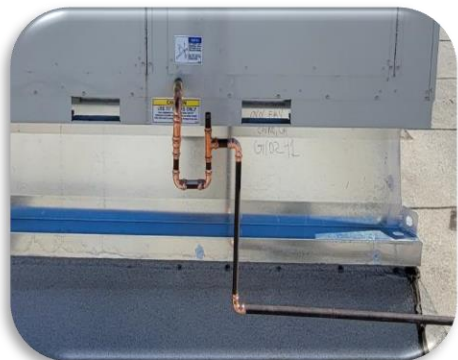
Copper P-trap Installed
