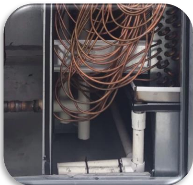
Upper to lower drain tube
