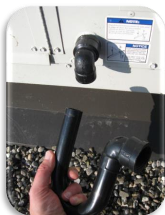
PVC P-Trap Installation
