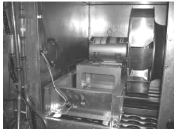
Figure 38 - 11-25 and 30 ton Supply Fan
