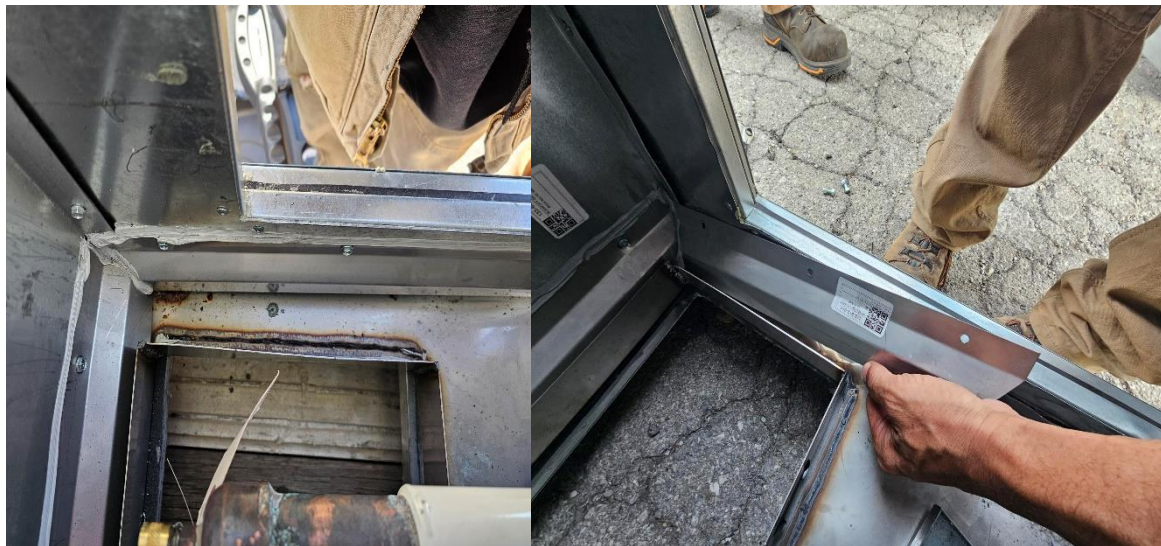
Fig. 8. Interior Coil Cabinet Panel Removal
